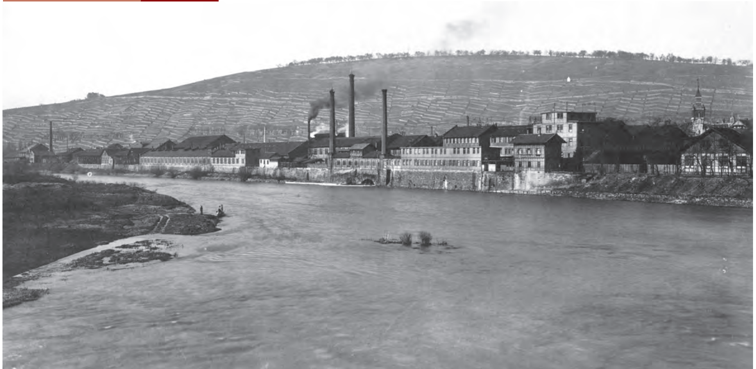
Factory halls of the Maschinfabrik Esslingen besides the station at the river Neckar in 1906. One can see the vineyards of the Neckarhalde in the background.
