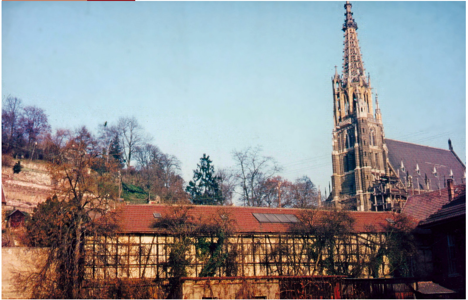
The Esslinger wine press on Mettinger Straße in 1970, shortly before its demolition (photo Paul Clauss)
