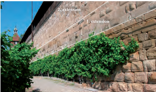
Shield wall at the covered staircase (Seilergang)
